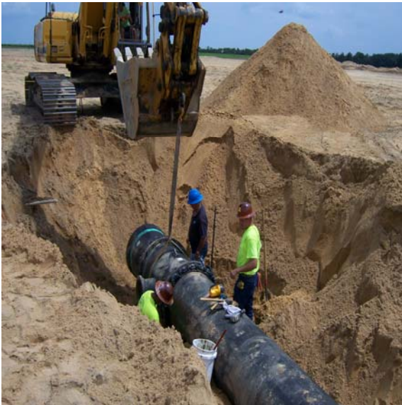
OCWS Pipe Fitters Install 30" DI Reclaimed Water Main
