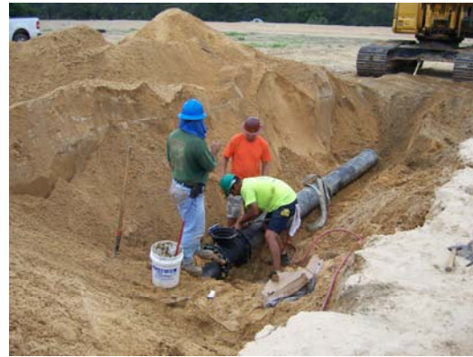
OCWS Pipe Fitters "Taking the Heat," for the Rate payers
