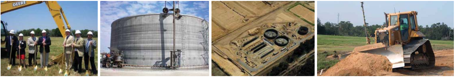
Okaloosa County officials decided to use three project delivery methods for the construction of a new sewage treatment plant — design-build, design-bid-build and self-performing the work.
