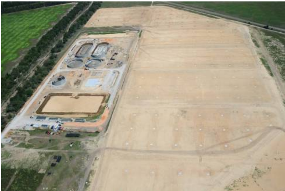
Completed Rapid Infiltration Basins
