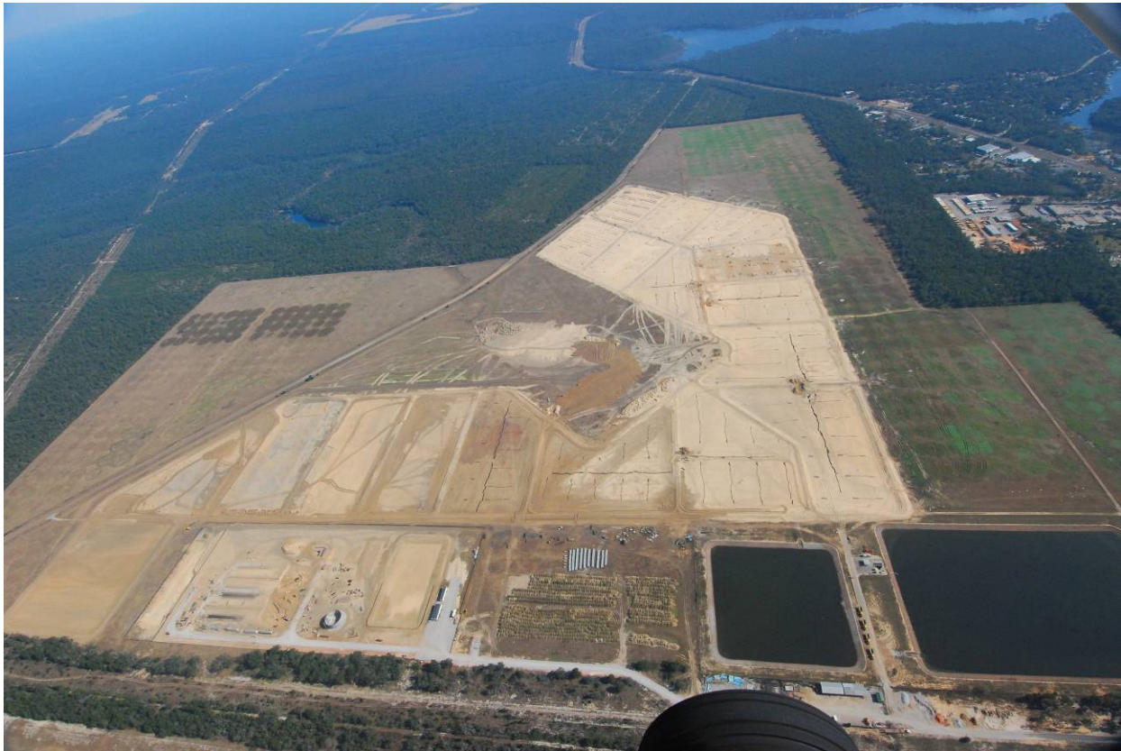
Garniers Spray Field, Arbennie Pritchett WRF and RIB Construction Site
