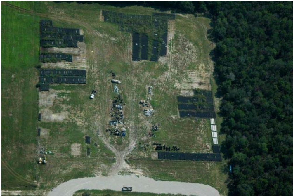
OCWS Material Storage Yard
