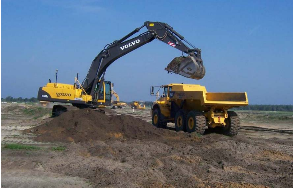
OCWS Construction Crews Excavating RIB Site
