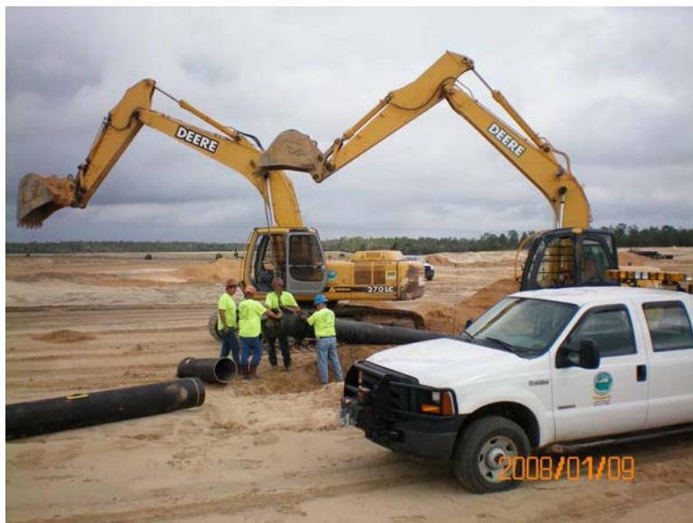
OCWS Construction Crews Placing RIB Piping
