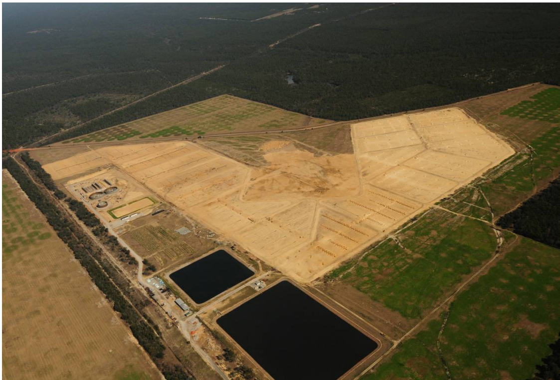
Water Reclamation Facility and Rapid Infiltration Basin Site Construction
